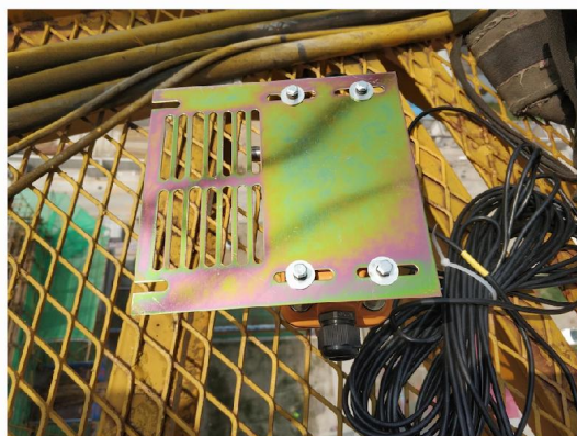
将传感器加装版固定好 First, install the sensors add plate
